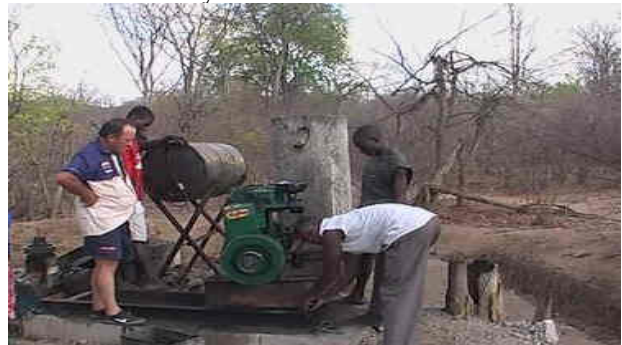
Johnny overseeing repairs to a pump.
